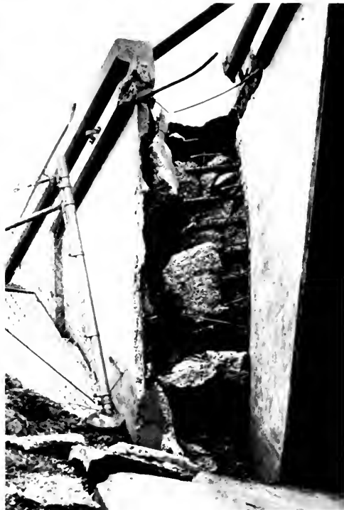
Photo 23. Damaged wing wall of abutment, Roxford Street undercrossing at Foothill Freeway [35].
